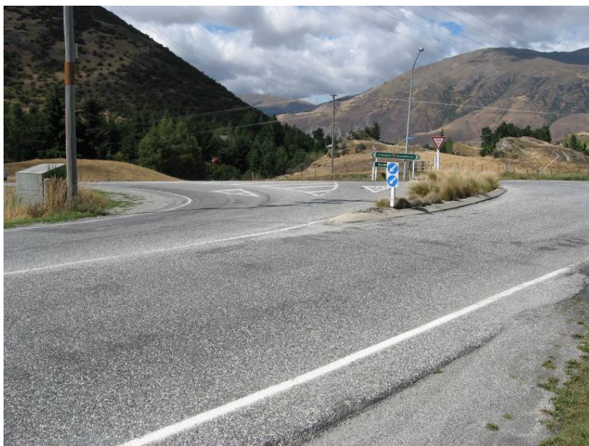
Photograph 7: Arrow Junction (State Highway 6 / McDonnell Road intersection)
