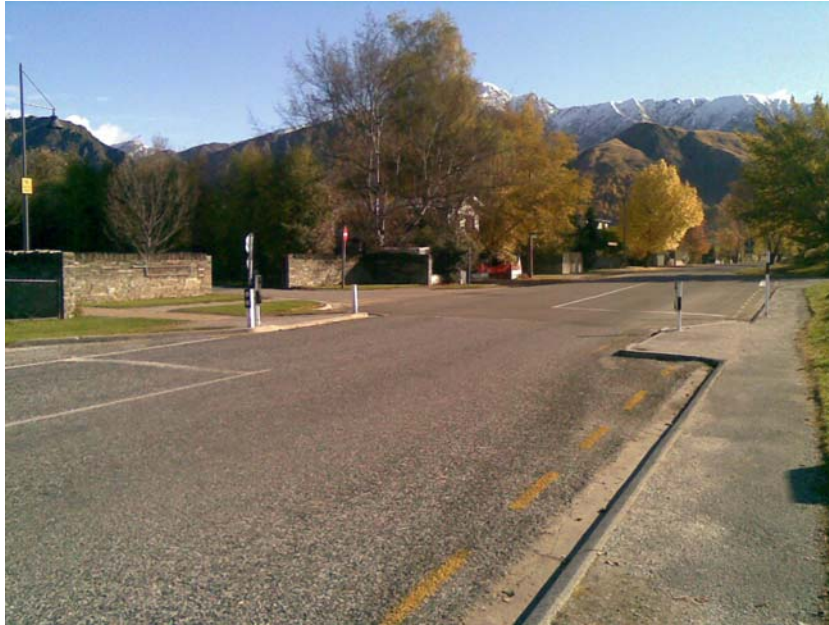
Photograph 4: Kerb build-out at school on Centennial Avenue
